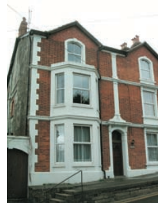
Victorian villas in contrasting brick and stucco detailing imposing building set tight against road frontage.
