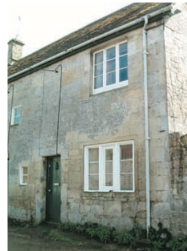
Simple two storey narrow fronted cottage. Simple detailing (originally would have had stone mullioned windows) building tight to pavement edge.
