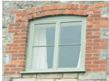
Simple brick window surround and arch detailing to casement window set in rubble stone wall.
