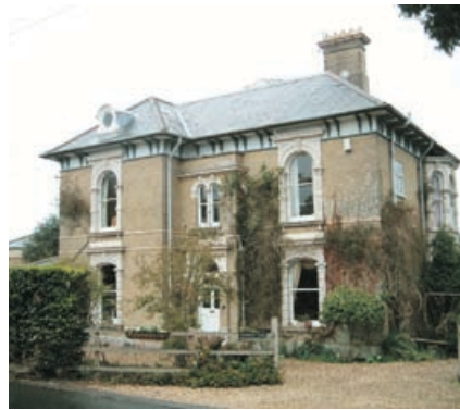
Large detached Victorian villa set back from street. Ornate classical window surrounds in stone. Use of buff brick as principal walling material is relatively rare.
