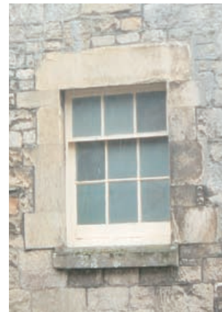
Sash window set within robust stone quoin surround.
