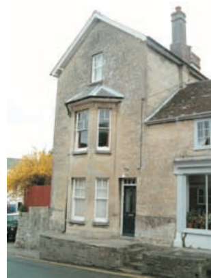
Narrow-fronted well-proportioned two and a half storey Victorian town house gable end to street. Two storey bay provides key feature to elevation in dressed stone.
