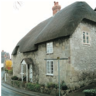
One of the relatively few thatched buildings in Tisbury. Simple cottage in rubble stone with casement windows. Building set back from street with small front garden.
