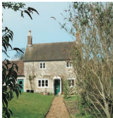
Detached stone cottage with plain clay tile roof. Simple detailing to openings and asymmetrical composition are attractive features.
