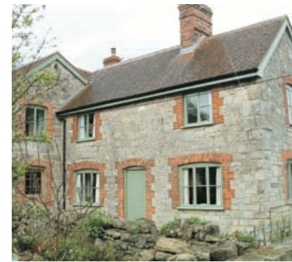
Brick window surround detailing to simple cottage which addresses lane gable on.
