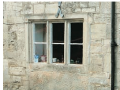
Medieval stone mullioned window to stone cottage.
